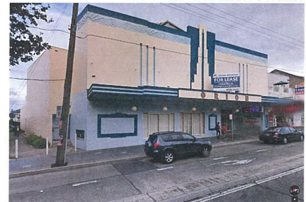
5 ORION CENTRE (HERITAGE) OPPOSITE SITE
